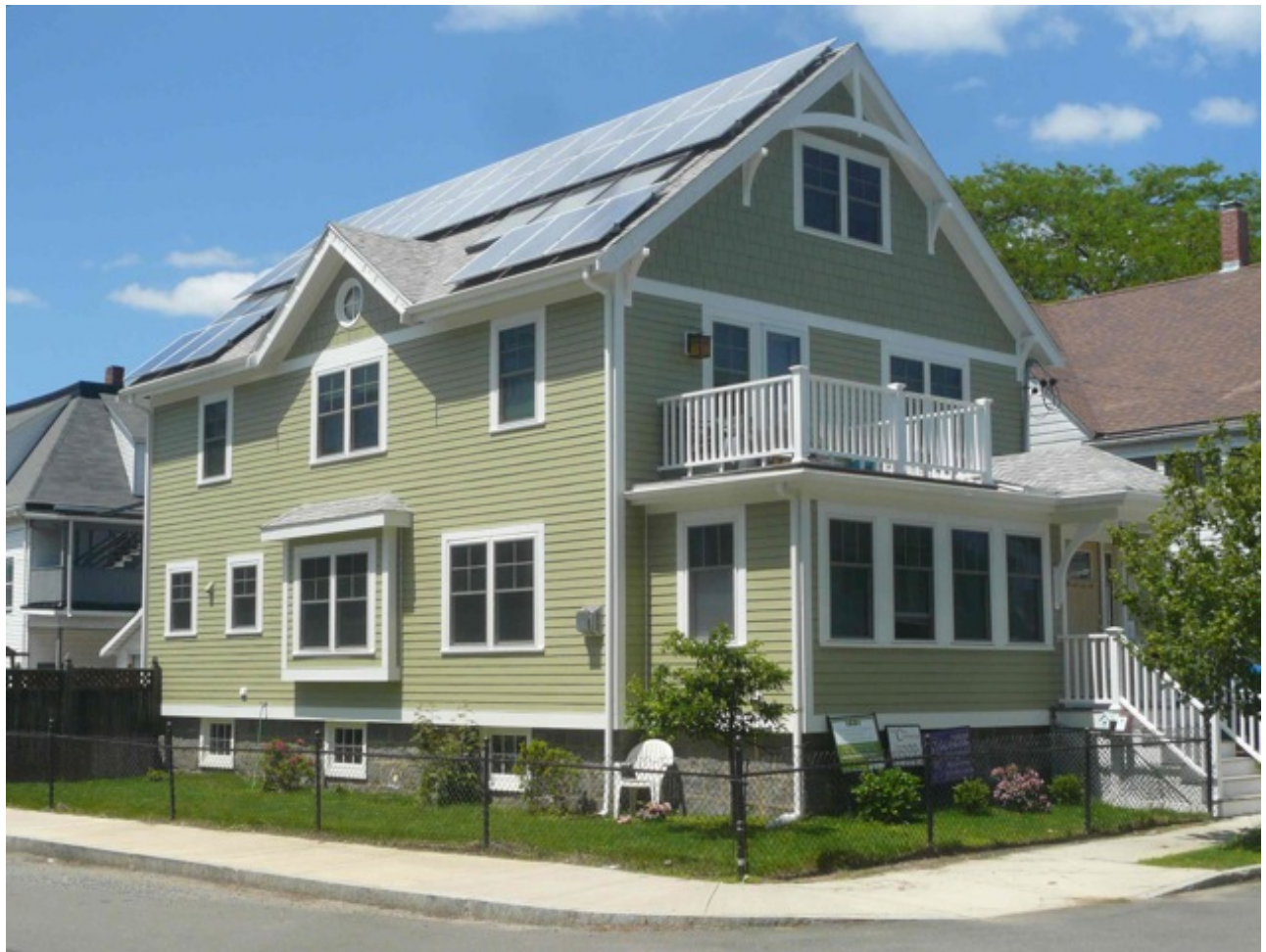
New 4-story home with super-insulated exterior wall and roof build-outs and south-facing solar installations.
